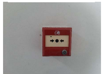
Fire Alarm Manual Station
