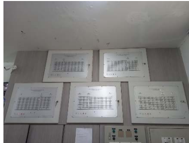
Graphic Annunciator Fire Alarm
